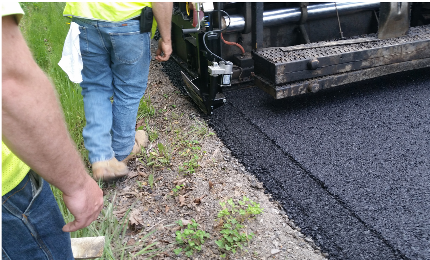
Willow Designs' safety edge systems are built specific to your paver to maximize efficiency. According to the manufacturer, the systems can be removed or attached in 30 seconds or less even while the paver is in full production. Originally designed to fit the Pennsylvania DOT specification that devices must be able to adjust the angle of the safety edge, Willow's system also offers a vertical adjustment to help with applications on thick lift courses.
