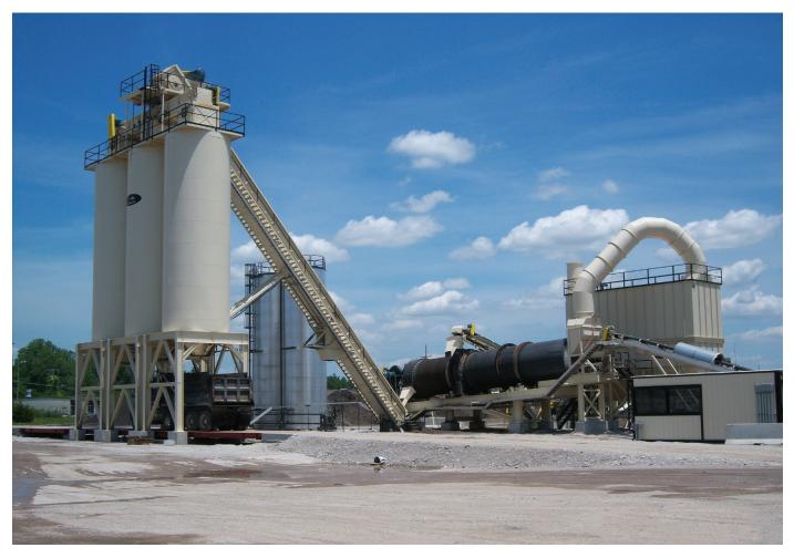
An HMA plant with an annual production rate of 100,000 tons emits in one year the same volatile organic compounds (VOCs) as two residential fireplaces during the course of one year and the same VOCs as a typical commercial bakery operating for two days.
